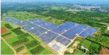
The 58MW Oriana Solar Farm in Puerto Rico. Pic: Sonnedix
